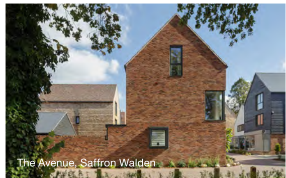
Figure 5.111: Gable end of house engaging with public realm
